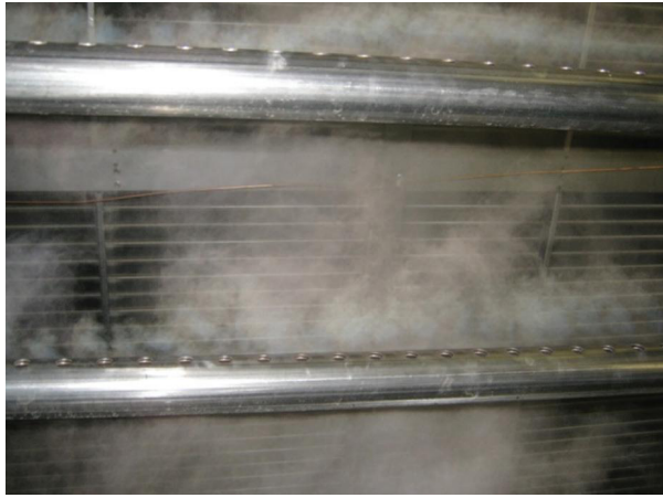
FIGURE 1 Uninsulated steam bayonet (left) and insulated bayonet (right).
