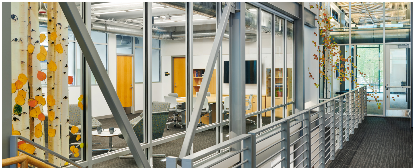
Top lighting and interior glass partitions integrate daylighting into the interior of the WELL Gold Aspen Police Department. (@Dallas & Harris Photography)
