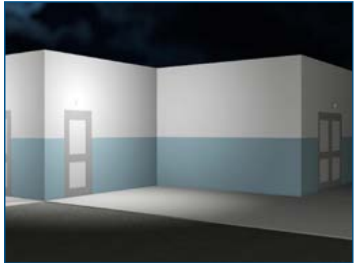
Figure 11 – White lights flash at doors nearest the danger.
