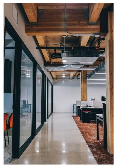
*Glulam was used for the beams, columns, and decking at 1040 W. Fulton in Chicago.*
