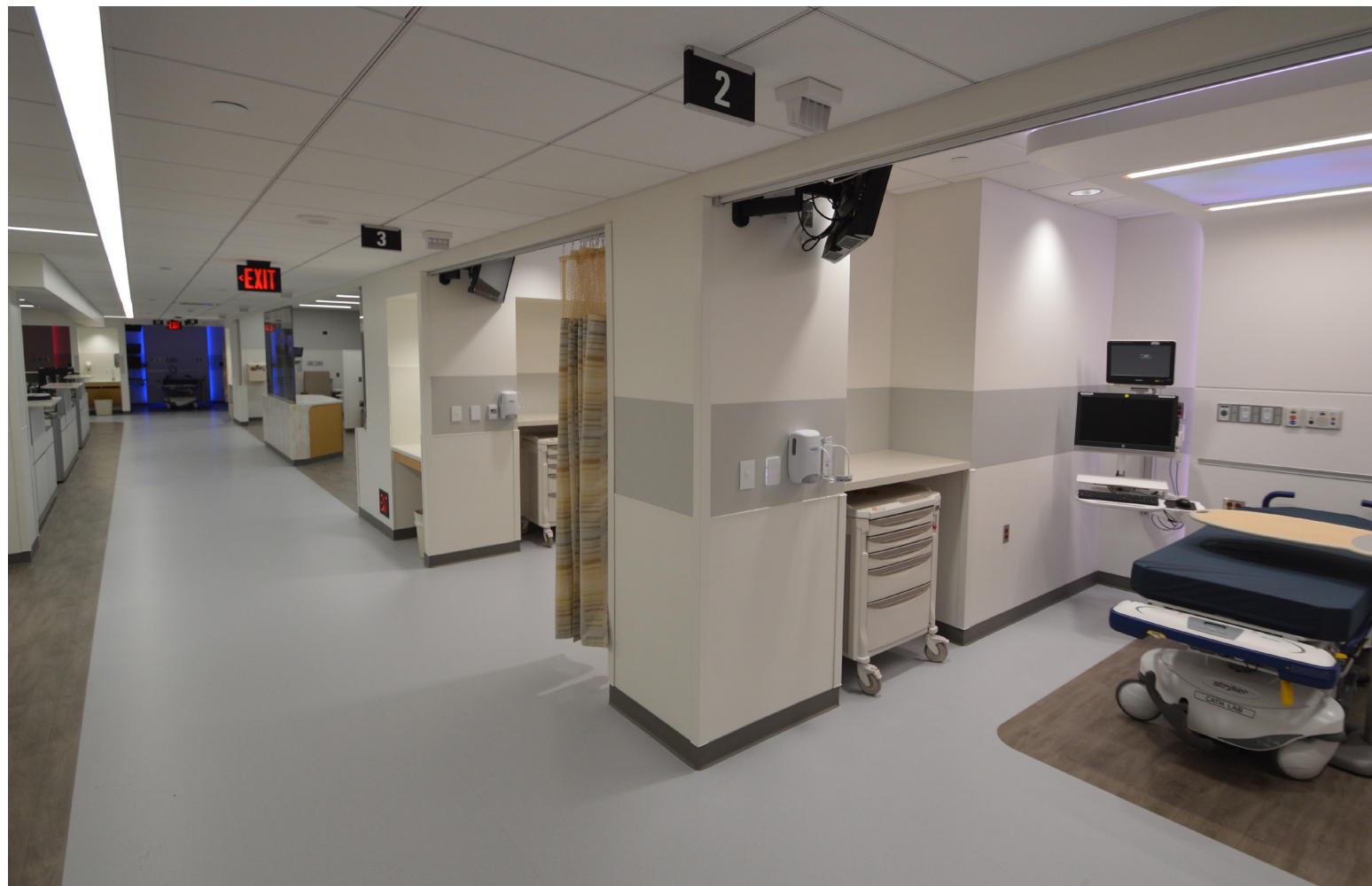
Prep and recovery bays in the cardiac catheterization lab at Advocate Lutheran General Hospital in Park Ridge, IL. The lab is part of the hospital's Heart Institute and is located directly below the emergency department, enabling quick transport in an emergency. The exit pathways lead to adjacent areas in the hospital.
