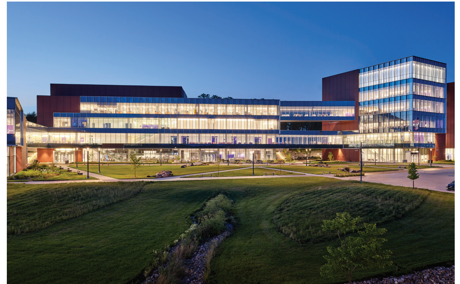
The all-electric Des Moines University Medicine and Health Sciences Campus is modeled to reduce operational carbon by 65 percent.
