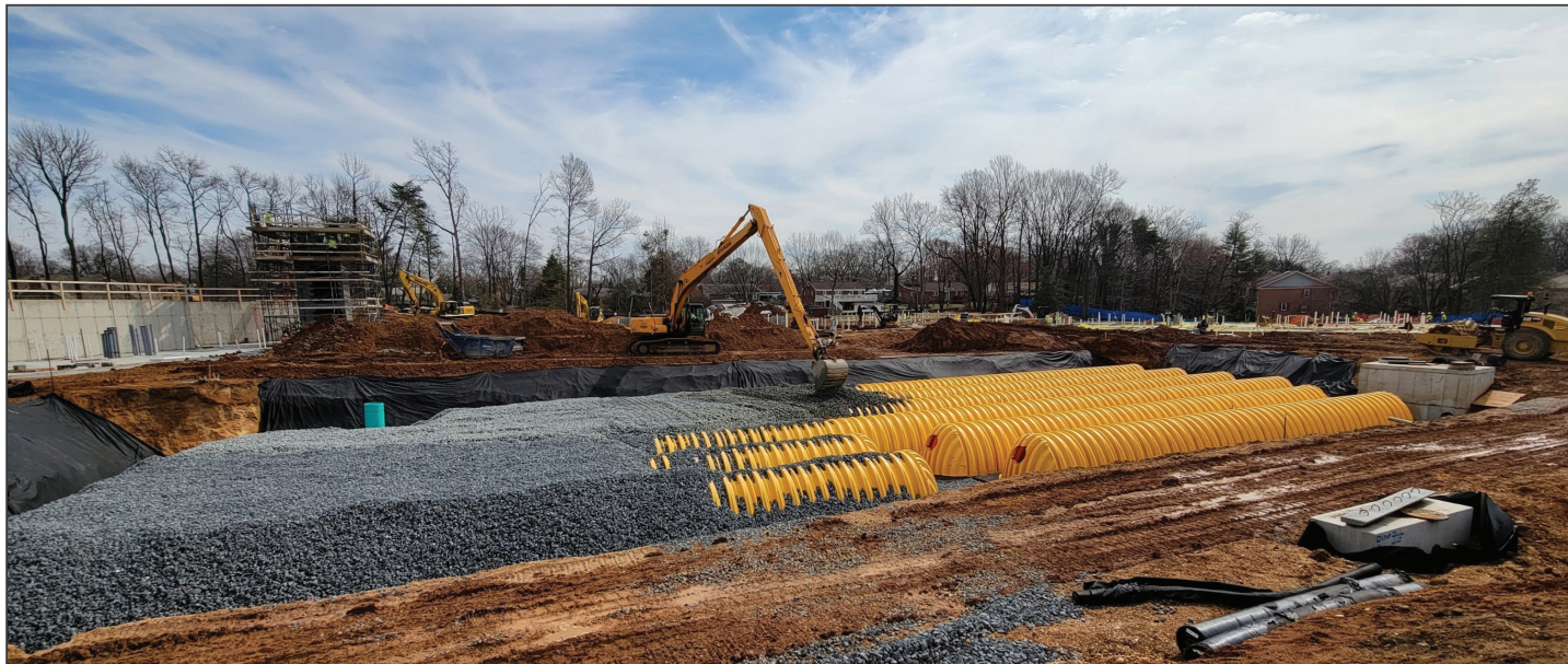
HDPE products provide a lower-embodied carbon option for piping and retention systems.
